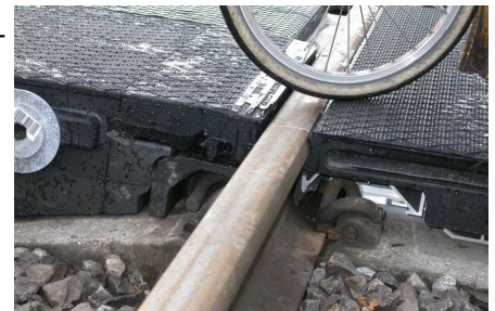
Safer rail crossing for cyclists and wheelchairs
